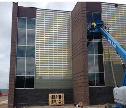
Park Center Senior High classroom addition
