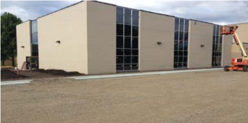
Osseo Senior High classroom addition
