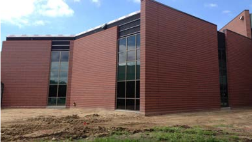
Maple Grove Senior High classroom addition
